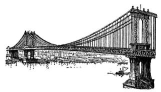
The last type of bridge is a suspension bridge. This type has a horizontal deck suspended from cables that are connected to tall piers. These bridges can span up to 7,000 feet in length. The Incas created suspension bridges made with rope before European colonization occurred in the 1500s.
